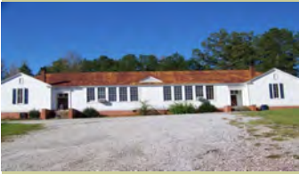
Woodworking Education Center 10544 Hwy 17, Maylene, AL 35114
